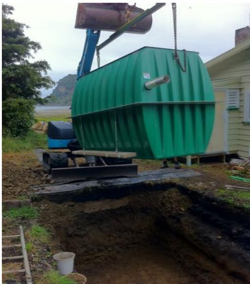
Because of the isolated location the system needs to be solar powered, this involves switching the standard pumps within the system with 3 phase pumps which draw much lower amperage. The cottage is rented as holiday accommodation, and with the system now fully installed it's almost ready for the influx of guests who will enjoy using the facilities over the coming months. This is another great example of a successful AdvanTex® wastewater solution for a remote and complex site.
