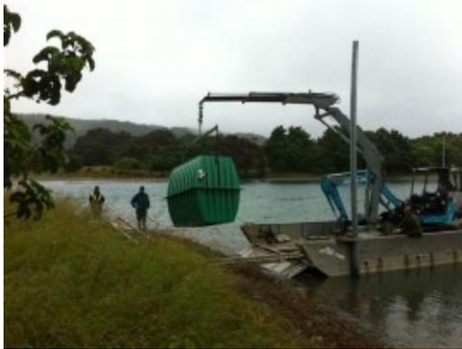
service the cottage. The first hurdle of the installation was arranging a barge to make the several crossings required to deliver the digger, equipment, and installation team, this was only possible at high tide which meant time management was critical. All excavations had to be completed at low tide and overseen by associated archaeologists who kept a watchful eye on each digger bucket load.
