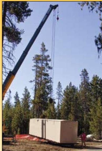
◀ This unit was installed at a state park in LaPine, Oregon. While AX-Mobile units are typically installed above ground, they can also be bermed or buried to grade.
